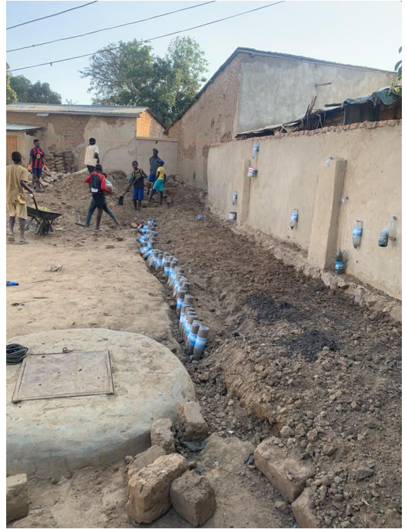
Drainage works and site preparation in progress.
