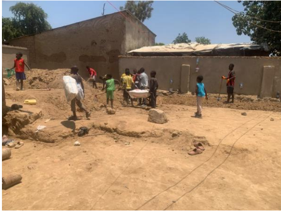
Community members working on the prepared project area.
